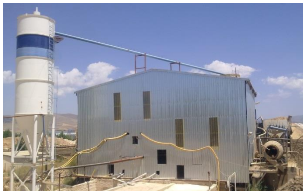
Fig. 12. Wastewater treatment plant belonging to the Baser barite beneficiation plant
